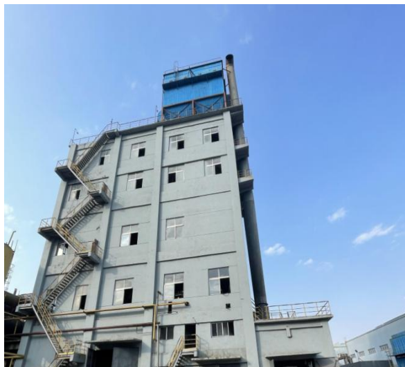
炼铁煤粉制备及喷吹粉尘
